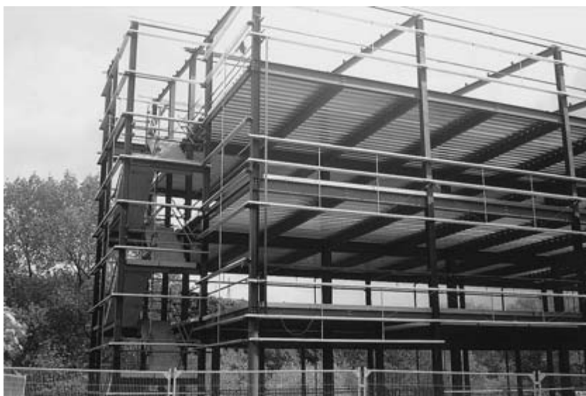
Fig. 22.1 Steel-framed office building under construction.
