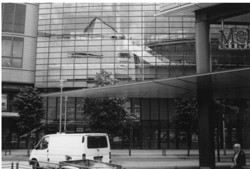
Fig. 23.1 Building with cantilevered canopy, Berlin.
